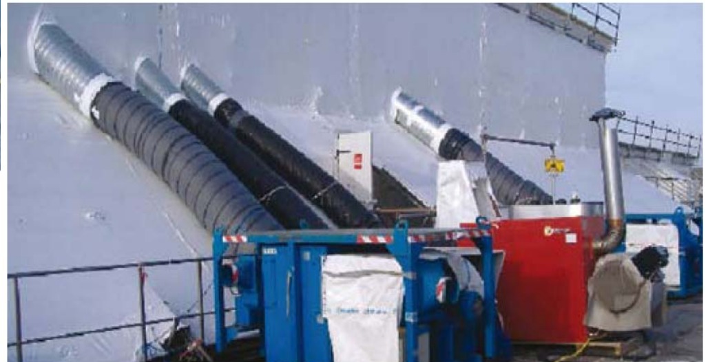
During repair the ship hull is covered by plastic foil to maintain a controlled climate. Dehumidifiers blow dry air into the covering, ensuring minimum corrosion between blasting away the old paint and applying the new.
