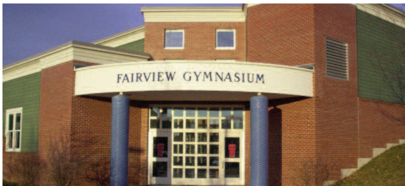
Fairview Elementary School had a serious indoor moisture problem that produced mold in classrooms and buckled an expensive gymnasium floor. Adding Munters' desiccant dehumidification equipment solved the problem.
