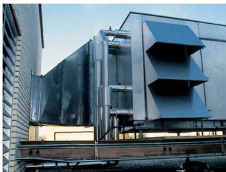
Figure 2. MedAire is installed at the make-up air inlet, avoiding construction interruptions to the HVAC system.
