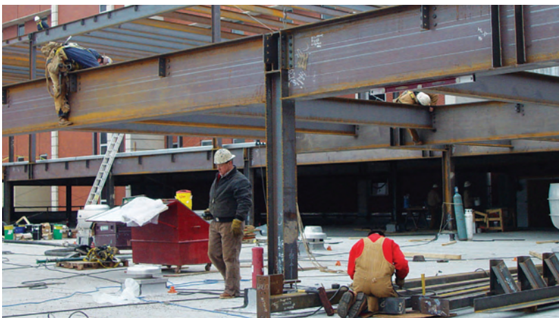
Construction teams renovated the St. Anthony Hospital in Oklahoma City. This project provided for doctors, staff, and patients advanced equipment and cutting-edge features in the hospital's facilities.
