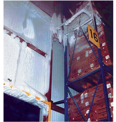
Left: Steve Cox points to a frost-free environment inside the Shaw's distribution center. Right: Before the installation of Munters DryCool equipment, frost build-up near exits formed blocks of snow and ice that threatened product quality, and forced workers to waste time chipping and thawing for hours every week.
